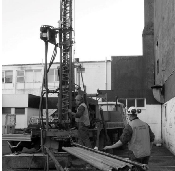
Figure 3. A drilling rig sampling soil to be tested in a laboratory.
